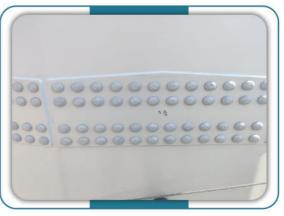
Vertical sections of the tower were previously filled with a special type of foam used during construction. The foam is squeezed into position as the steel plates are forced together. Due to tower oscillations the foam was uneven in places resulting in gaps where water was able to pass through and penetrate the interior.
