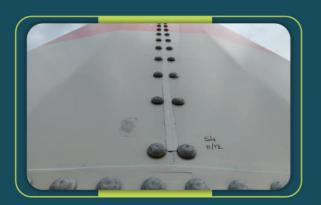
The solution for this was to remove any protruding foam from the vetical seams. We would then clean the area thoroughly, again to promote adhesion of the specially designed sealant tape.
