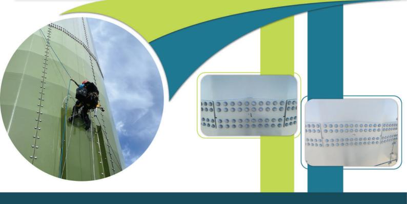
In total there were 11 segments. These varied in number of panels as there were more at the bottom and reduced nearer the nacelle. There were x24 horiztonal cover plates on each segment resulting in a total of 264 horizontal cover plates being sealed. There were 98 vertical seams on the tower which resulted in a total of 1078 metres of taping to be applied.
