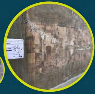
x4 separate structural laminations were applied to the affected area to rebuild the layers that had been removed. These extra structural laminations were necessary due to the incorrect removal of the spoiler. Cuts were found in the outer fiberglass layers which had been filled with paint. Due to the nature of these cuts being at varying angles causing structural stress' across the area these were removed.
