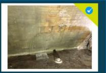
Cover laminate applied in order to spread the load over a greater surface area and to encompass the webfoot and web reinforcements.
