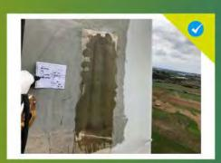
Additional fiberglass was layered over the top of the structural laminations in order to spread the load across a greater surface area. This was completed in order to reinforce the original defect.
