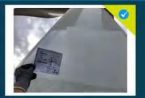
Upon completion of the laminate, the area was filled using sacrificial laminate and filler to restore blade profile. Filler then sanded and painted.
