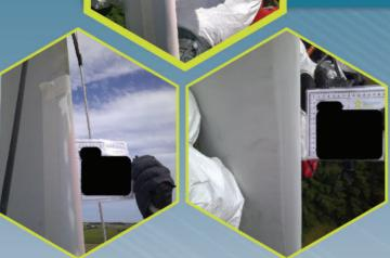
Damaged filler and paint were removed and replaced with a stronger brand of filler and repainted with a 2K paint. Small additional damages were found during the scheduled repairs. We consulted with the customer and we were able to complete these on the same visit.
